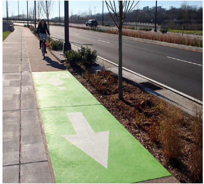
Figure 5.33 Raised bike lane example from Nashville, Tennessee
