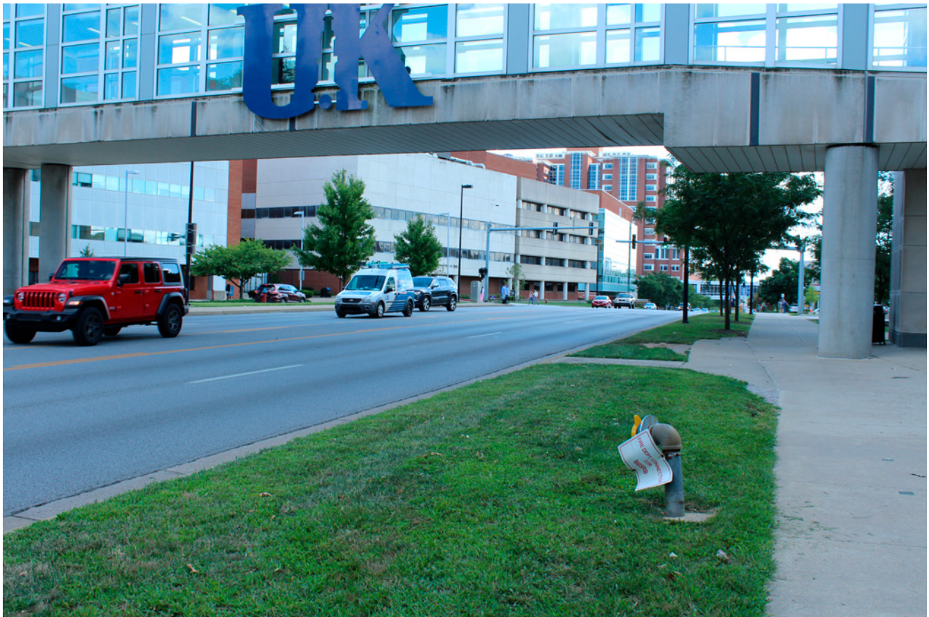
Figure 5.66 S. Limestone near the Medical Campus looking south
