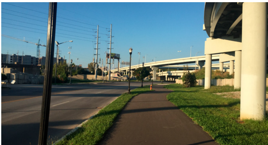
Figure 5.7 An example asphalt shared-use path in Louisville, Kentucky
