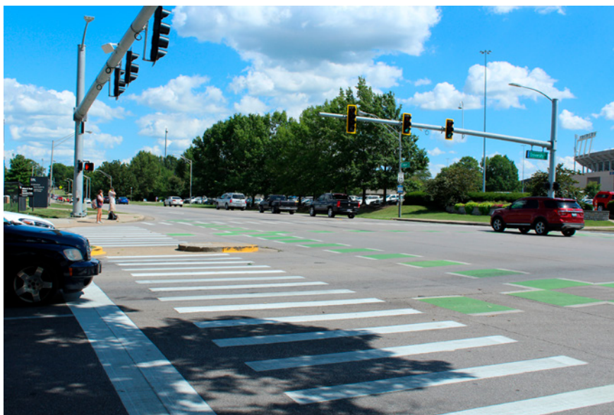
Figure 5.40 Example of enhanced green bicycle crossing at Cooper Drive and University Drive
