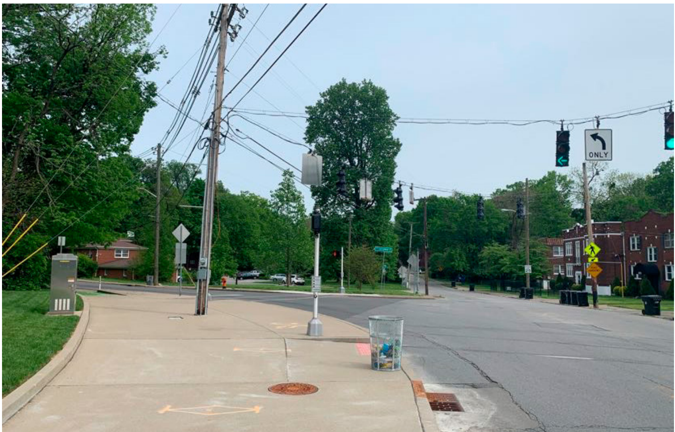
Figure 5.15 Urban, curbside shared-use path example in Louisville, Kentucky
