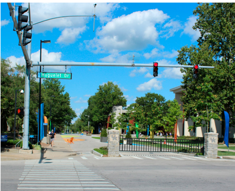
Figure 5.17 Huguelet Drive and Rose Street intersection and controlled access to the bicycle and pedestrian plaza
