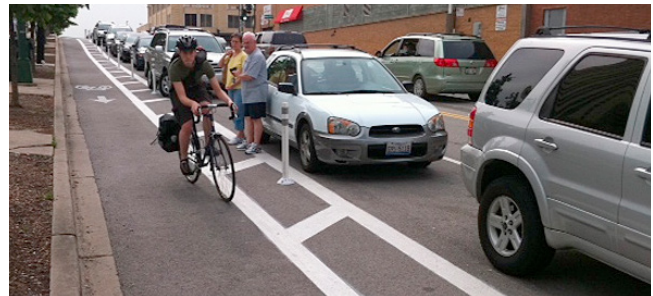
Figure 5.22 Example of a parking-protected bicycle lane in Chicago, IL (Source: NACTO)
